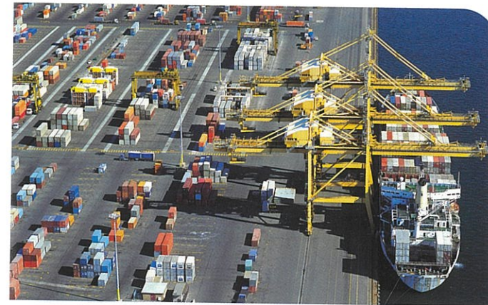
8.20 Modern dock facilities and containerised cargo have contributed to the growth of world cargo movements.
